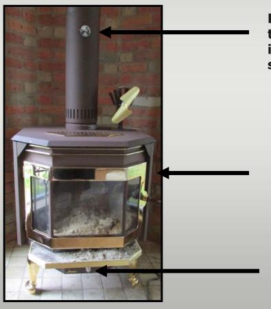
Reading of chimney thermometer installed 18 inches from the top of the stove
