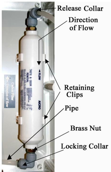
Then you need to release the nylon pipes from either end of the filter. Procedure:
