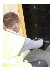
Mark hole positions – drill holes and insert plugs to suit 6 x 50 screws ensuring that the Wall Post is compressing the EDPM Pad
