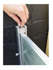
Once all panels have been pushed down so that they fully engage with each other, the Compression Blocks can be inserted and their bolts can then be finger tightened – do not use any tools at this stage.
