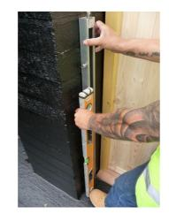
Use packing shims (normally for double glazing) easily available from Builders Merchants - so if narrow at bottom, pack out at top – if narrow at top pack out at bottom
