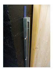
NOTE: The Vertical D-Seal is supplied so that it 's position is retained, so that it is longer than the Wall Post. This is to ensure that when the Wall Post is positioned onto the EPDM Pad the D-Seal will also seal into the Pad
