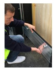
The first (Bottom) panel is lowered into position, ensuring it is correctly positioned with the thicker Dual Hardness seal at the bottom of the panel.
