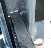
It is important to check that both ends of the Middle Seal extend completely to either end of the panel. If they are short of the end there is a chance that they will not seal to the vertical D-Seal on the Fixed or demountable Post.
